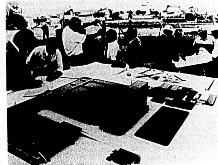
Barilla Builds New Plant. The world's largest plant for production of pasta is under construction at Corte di Pedrignano, on the outskirts of Parma. The plant, a model of which is shown in the foreground, will have an area of 60,000 square meters (645,000 square feet), and is being built for Barilla S.p.A., one of Italy's leading food-product manufacturers. It is located on a 1.2-million-square-meter (295 acres) site on the Autostrada del Sole, one of the main Italian highways.
